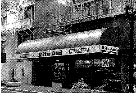
Out of scale canopy made of poor quality materials that serves primarily as signage
