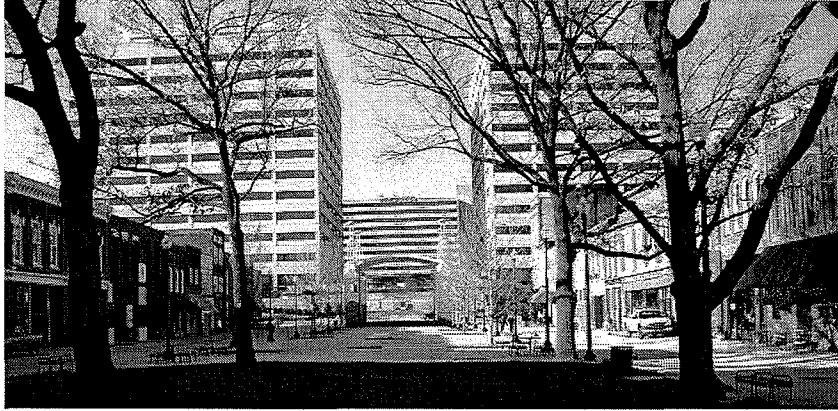
Unconnected, discontinuous, overly wide pedestrian-only walkways
