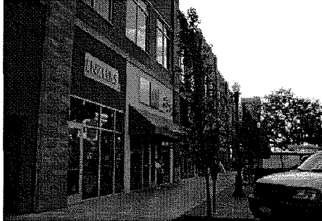
Glazing with simulated divisions that do not connect the sidewalk or street to the interior
