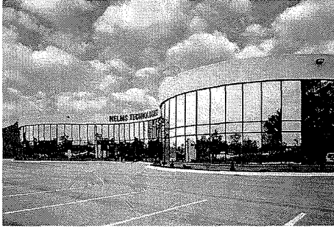
Unarticulated roof lines
