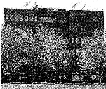
Rooftop telecommunications equipment visible from public spaces
