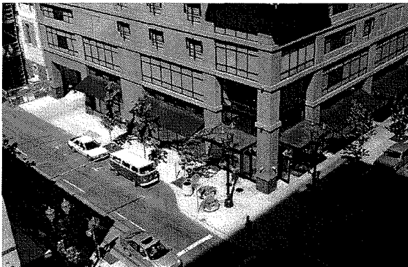
Parking garage design resembles mixed use development, limits driveway opening and integrates
